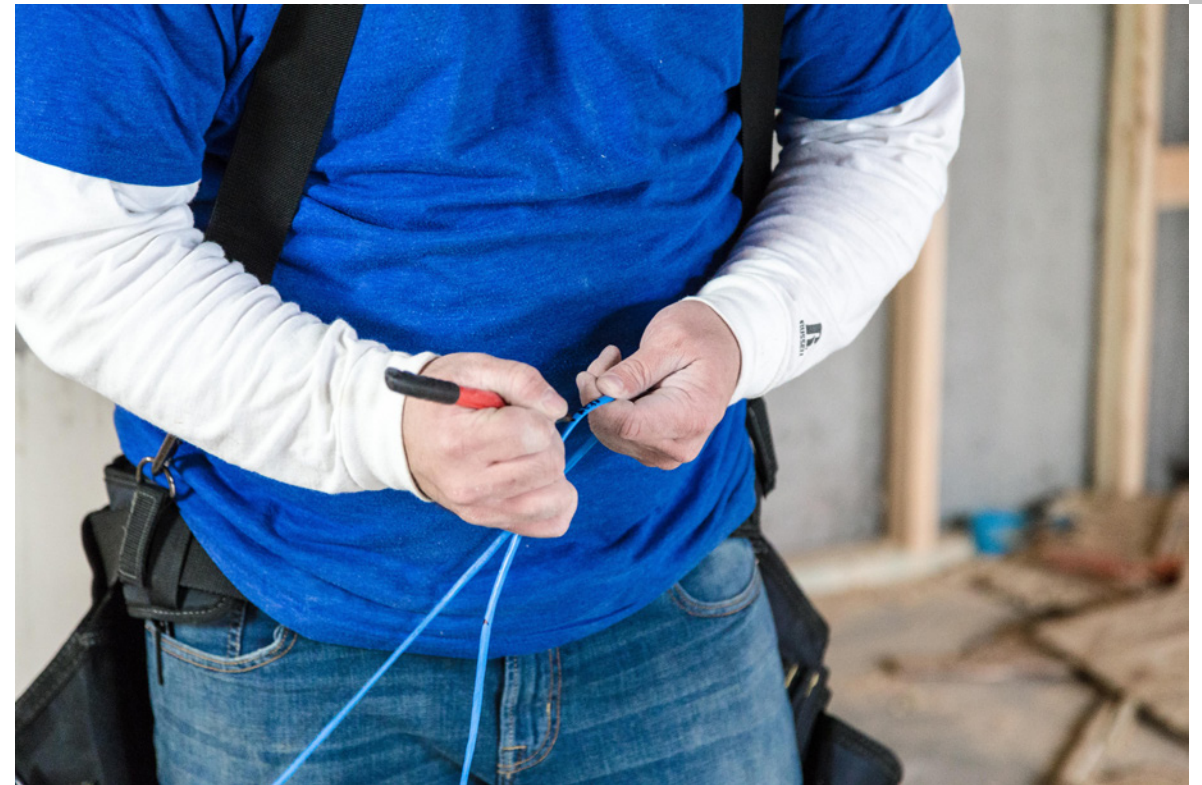
Label each wire a few inches above where you plan to cut.
