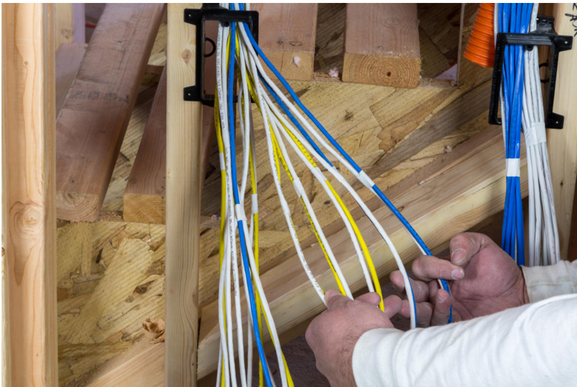
Keep TV's Bundled together. I tape the (2)Cat6 for Video Distribution together, and the additional (2)Cat6 for Control and Network together.
