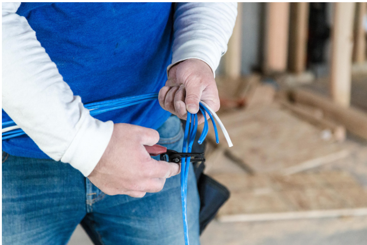
Only after labeling, cut the bundle to length.
