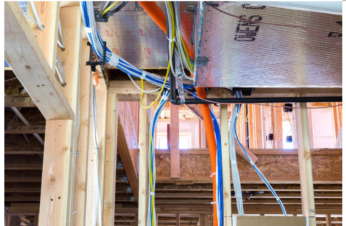
Low voltage brackets (mud rings) for cable management.
