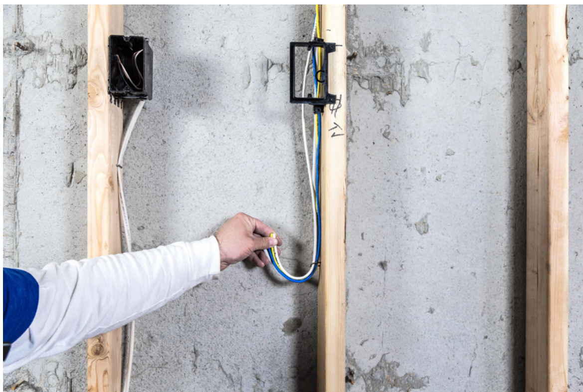
Finished TV drop ready for insulation and drywall.
