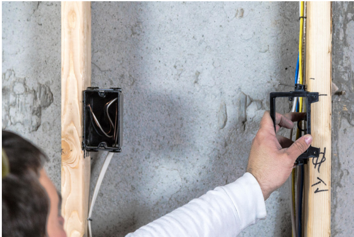
Staple the cable bundle several inches above and below the low voltage bracket.
