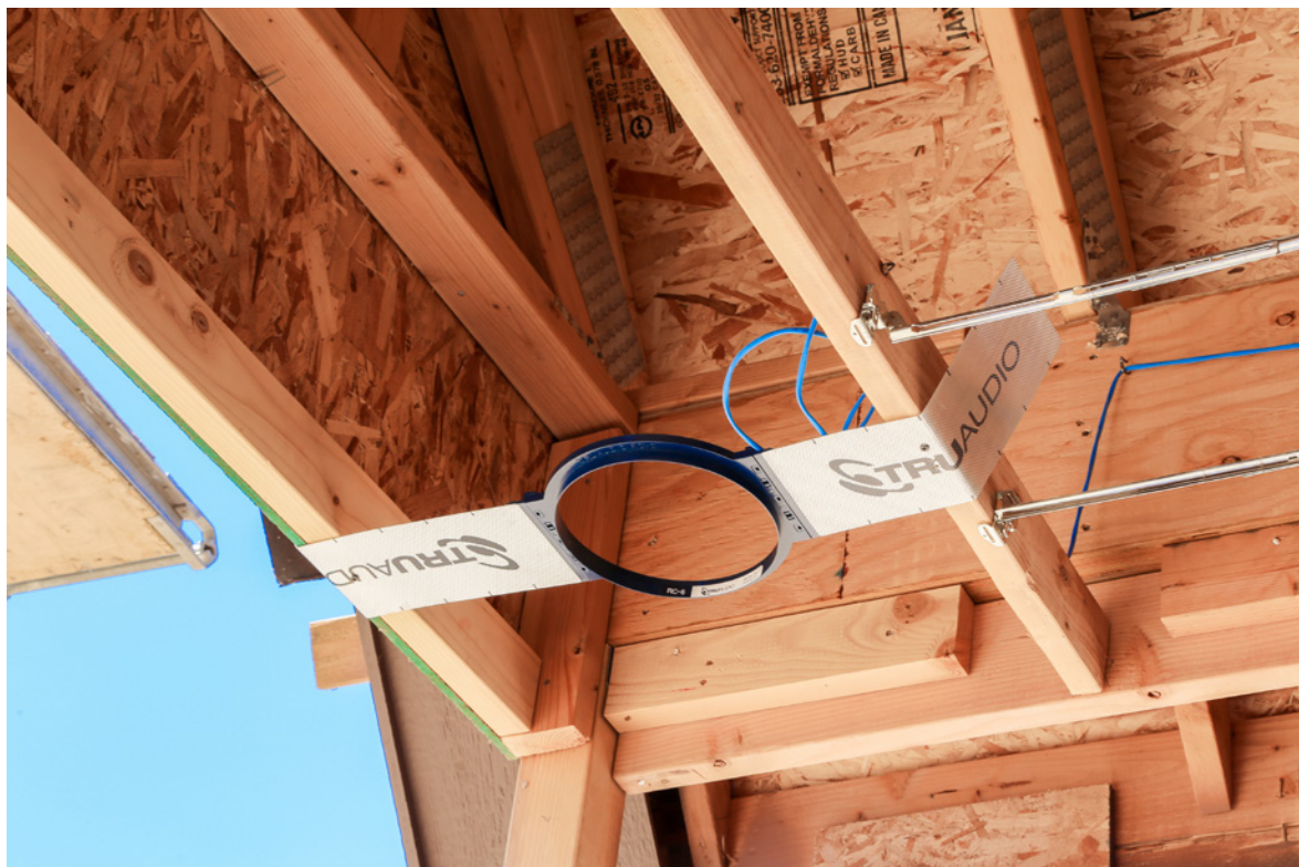
Outdoor audio prewire with speaker ring.
