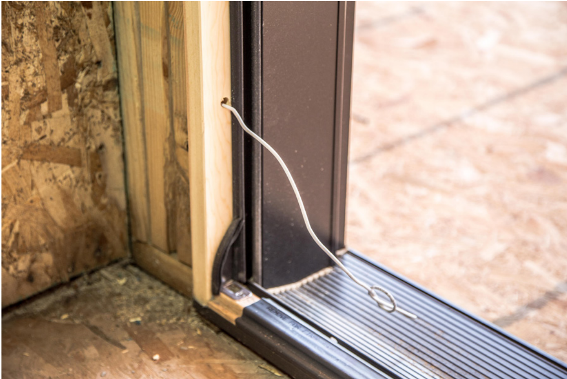
Wire shown for a 3/8" door sensor.
