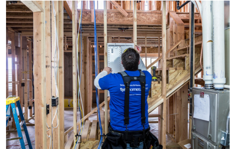
Place the low voltage panel(s) at equal height with the electrical panel(s).
