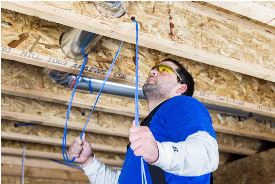
Gently pull the cable to the mechanical room..
