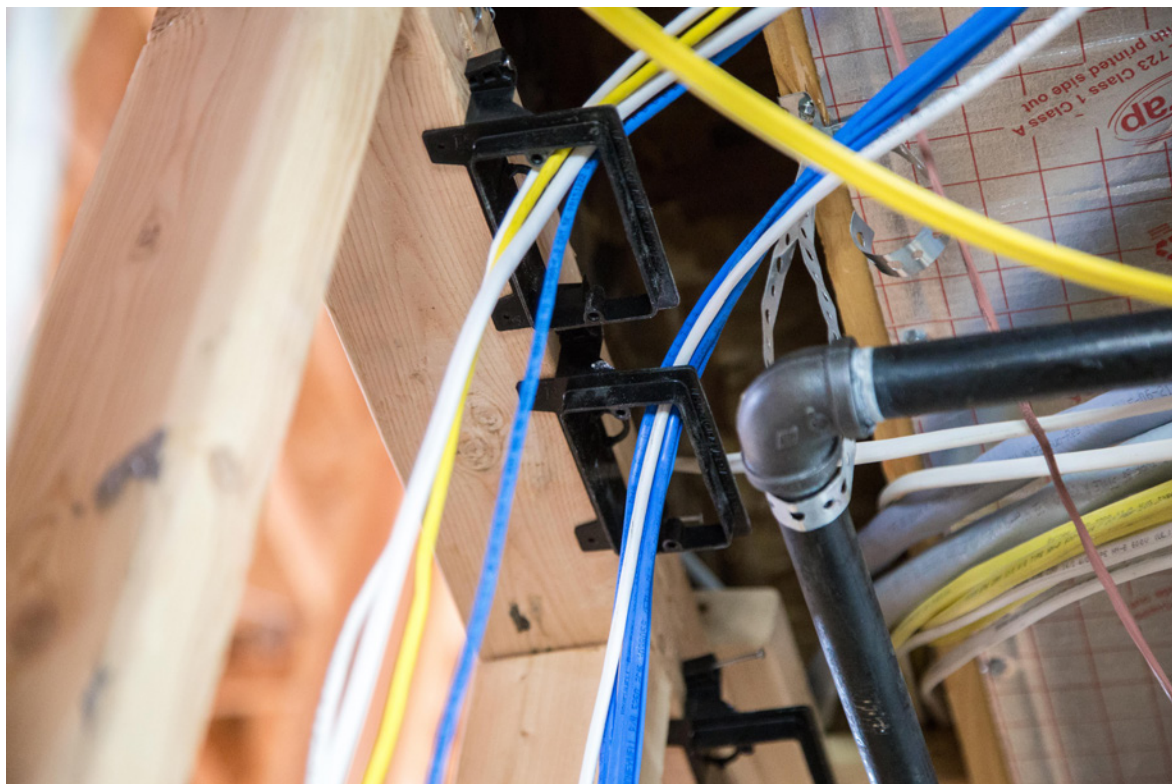
Low voltage brackets (mud rings) can help with cable management.
