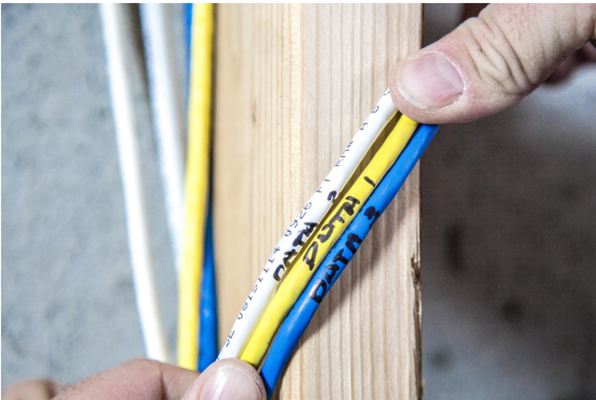
Labeled cables/wires.
