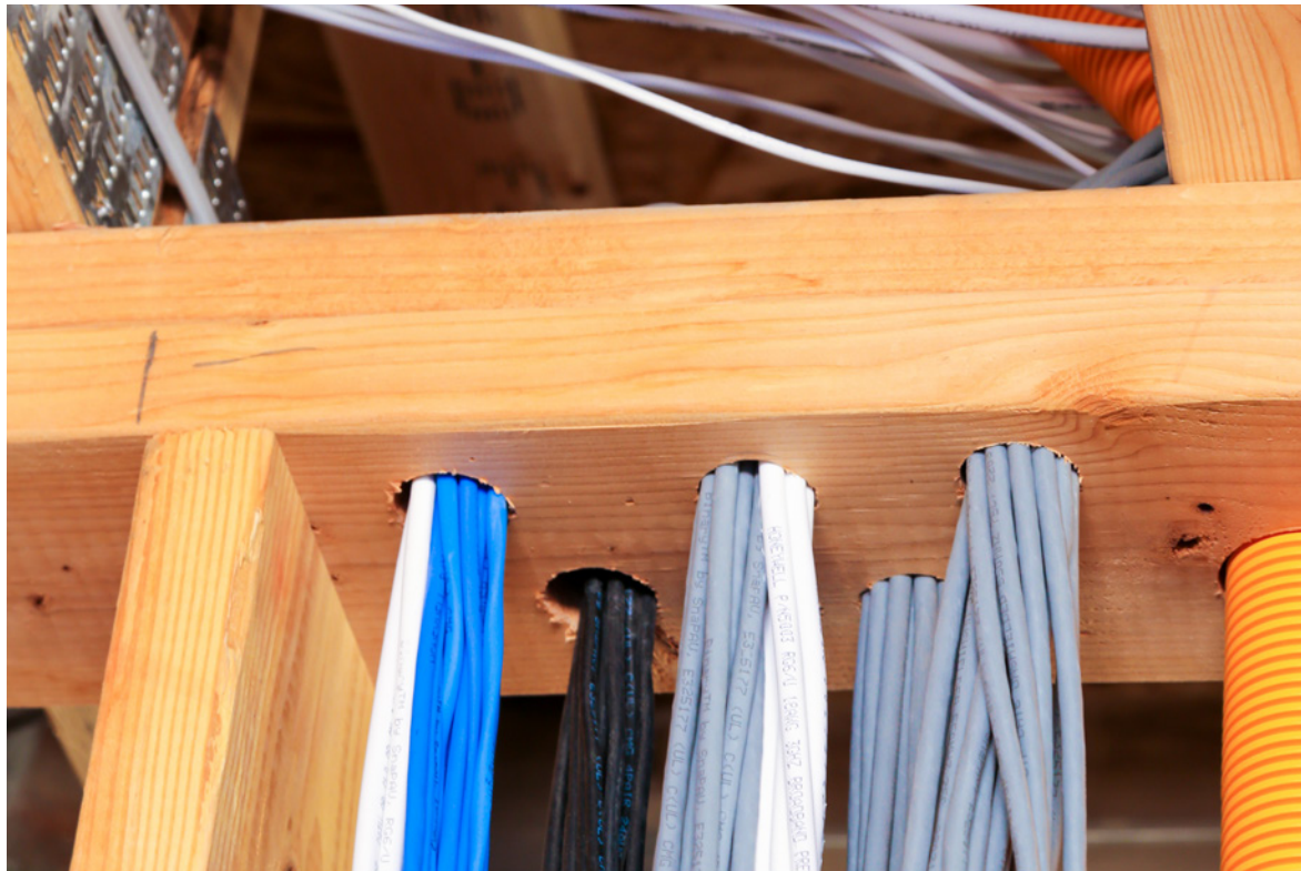
Multiple holes make for easy organization during prewire.
