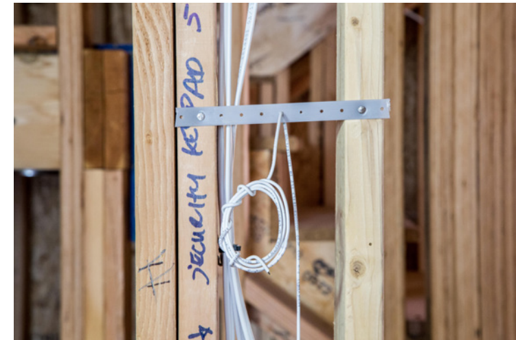
Keypad prewire held with hanger strap.
