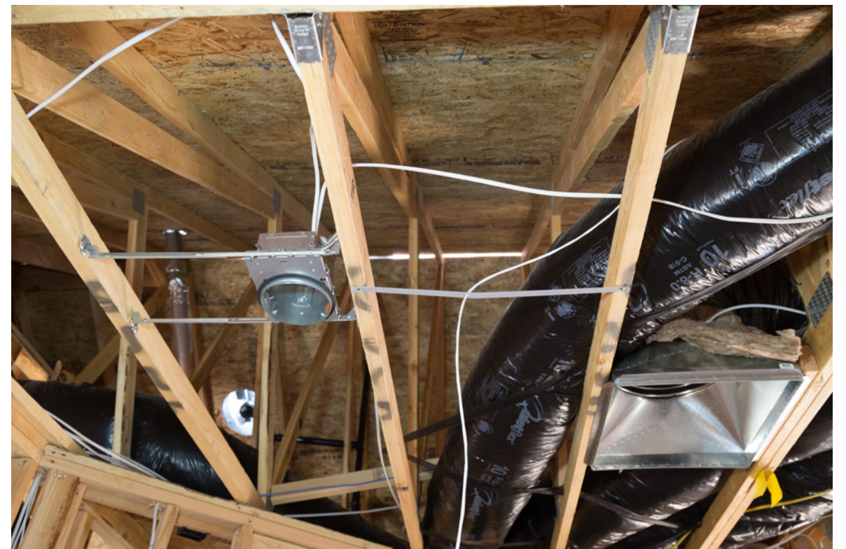
Audio prewire with plumber's strap.
