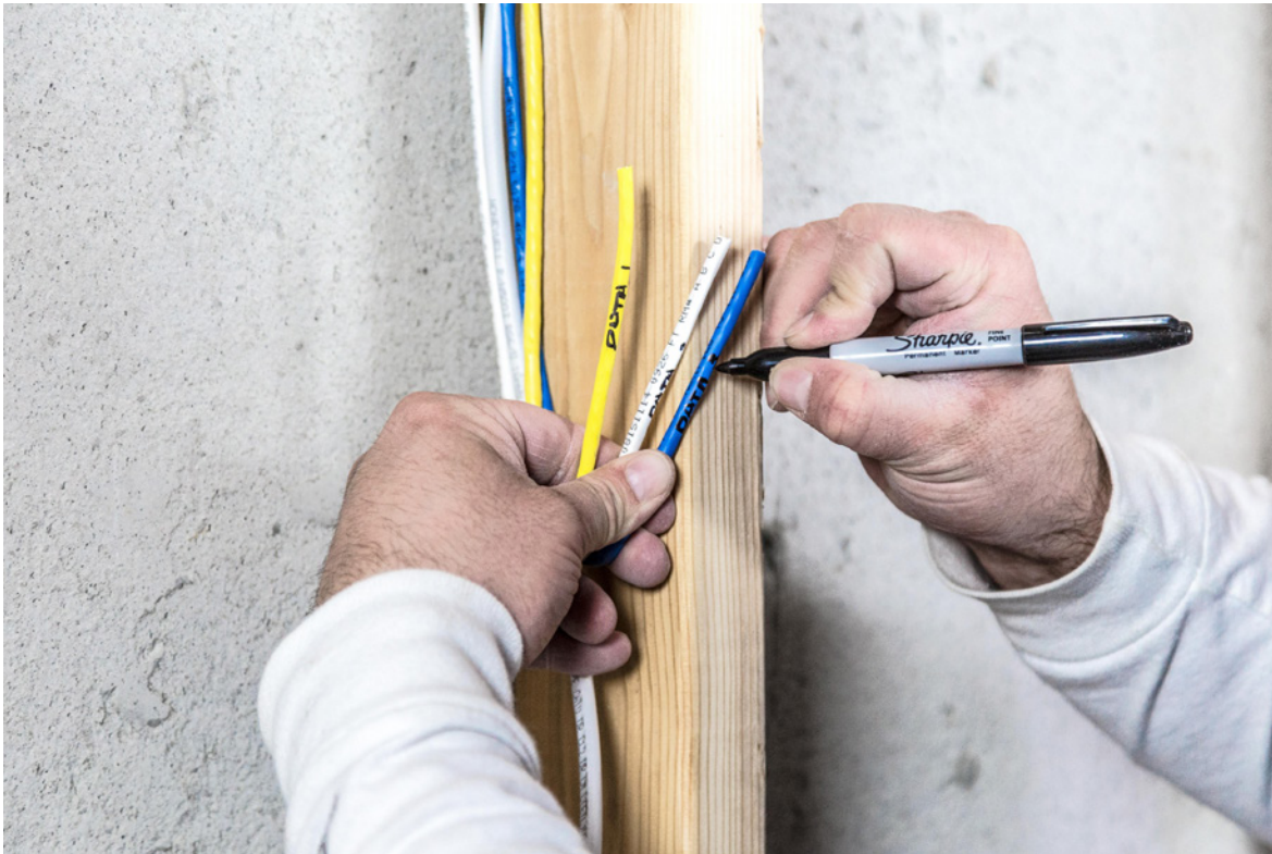
Label the trimmed end of every cable/wire.
