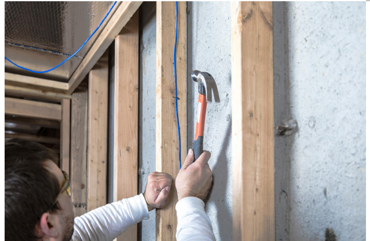
Gently staple the wire. DO NOT crimp the wires.
