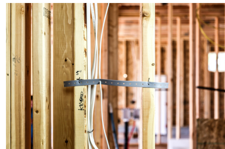
Keypad prewire held with hanger strap.
