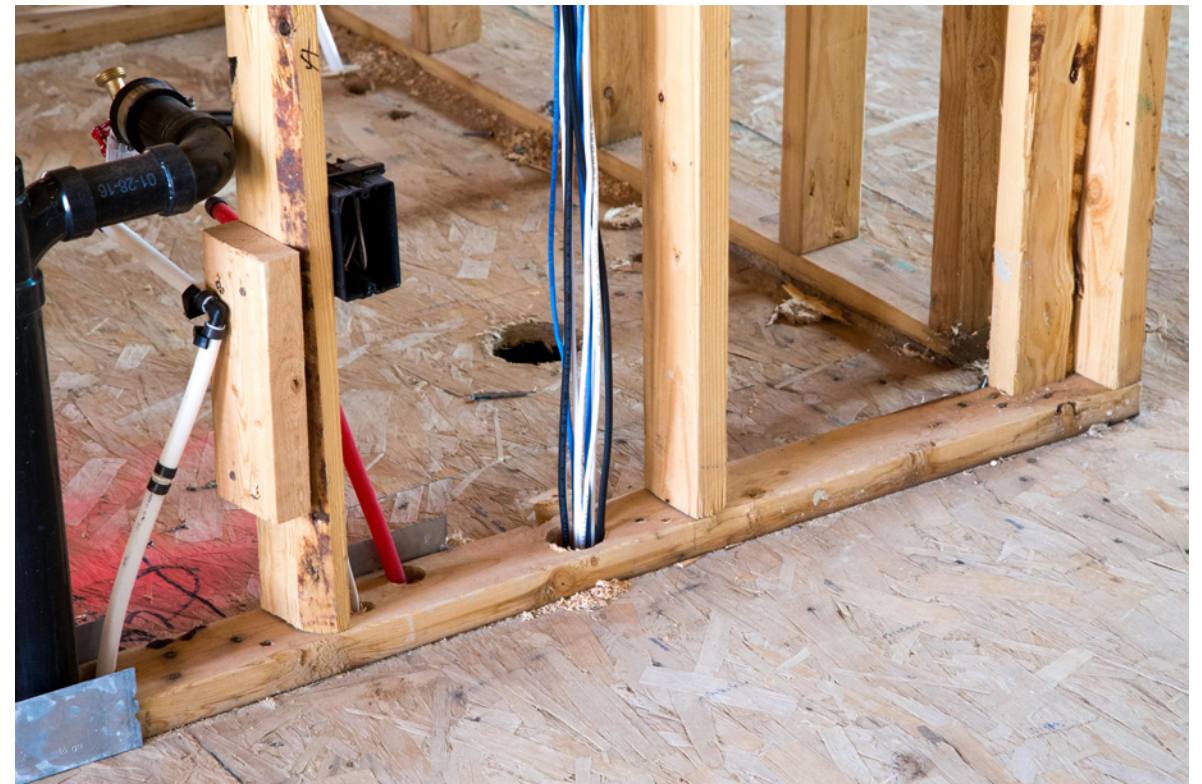
Drill a clean hole for runs between levels.
