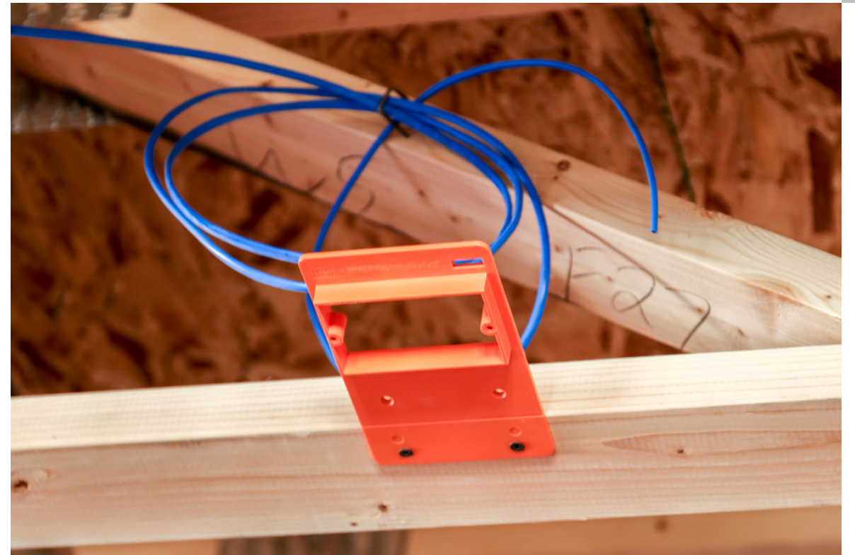
Special Single Gang Bracket, sits away from stud 1", and breaks away at install
